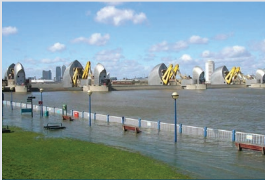
The 100th closure of the Thames Barrier. Although there is localised flooding downstream, the city behind is protected.
